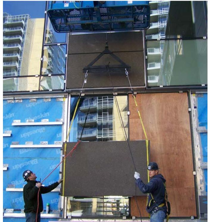
*Top:* Stainless steel prestressing enables thin, durable lightweight panels. *Left:* Stainless steel connectors permit fast installation on building exteriors. *Right:* A number of lightweight ARCIS panels can be shipped on the same truck to reduce transportation costs. *Far right:* Rainscreen panels can be installed with a minimal crew and a small crane or lift.
